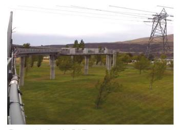
Figure 5 - John Day After Full Flow wide view The John Day Full Flow system is elevated about 75 feet above the ground.
