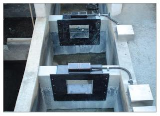
Figure 2 - All fish ascending the ladder must pass through these antennas.
