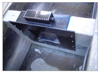
Figure 1 - A close-up of one of the PIT tag antennas installed in the fish ladder at Roza Dam.
