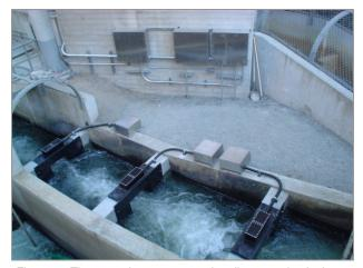
Figure 3 - There are three antennas, in adjacent weirs, in the adult ladder at Roza Dam.
